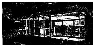
Shubin + Donaldson Architects Carpinteria Guest House Carpinteria, CA 56
